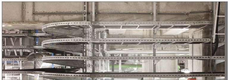
Attachment of cable support systems
