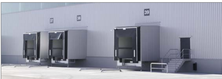
Attachment of profiled metal sheets on the walls and roof
