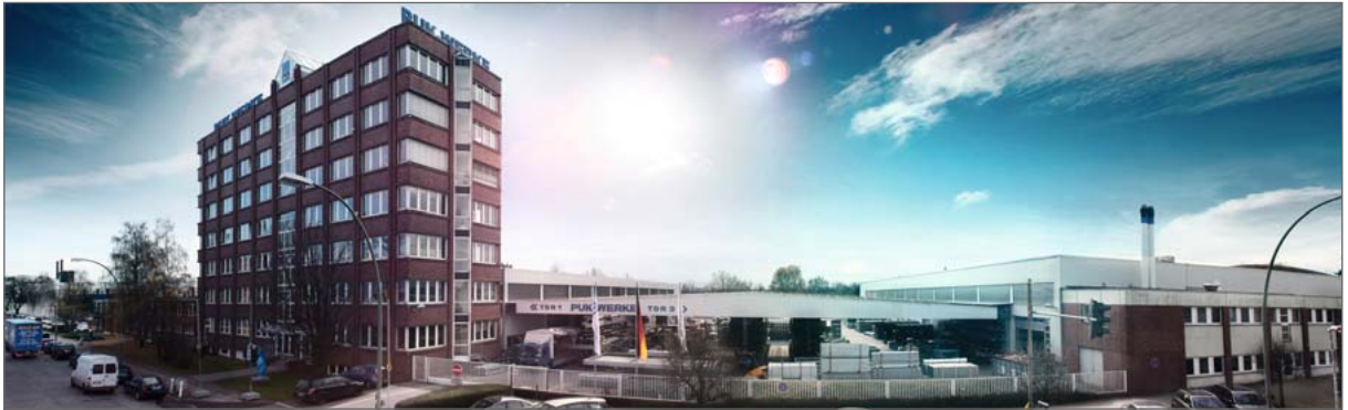
JORDAHL's registered office and administrative headquarters on the premises of its affiliate PUK
