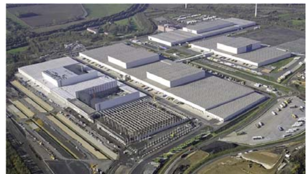
Connection to roof
