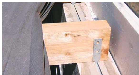
Joist attachment to ring beam with timber fixing straps and brick tie channels
