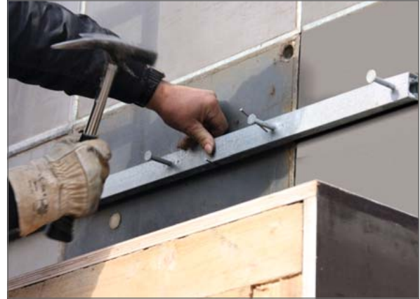
Nailing the anchor channel to the wood form
