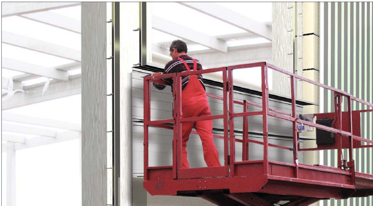
Installation of a multi-layer insulated corrugated metal siding wall
