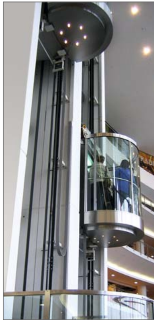
Attachment of elevator guide rails
