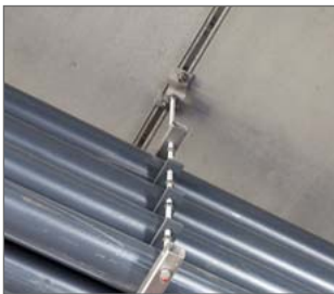
Attachment of pipe-work
