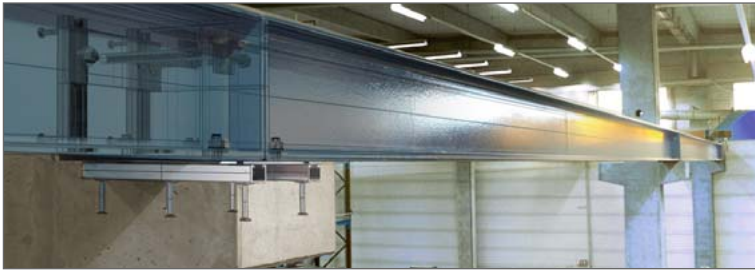
Attachment of crane rails to prefabricated concrete elements
